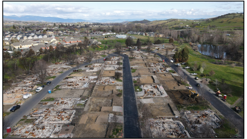
Ash and debris removal in the Archie Creek Fire area
