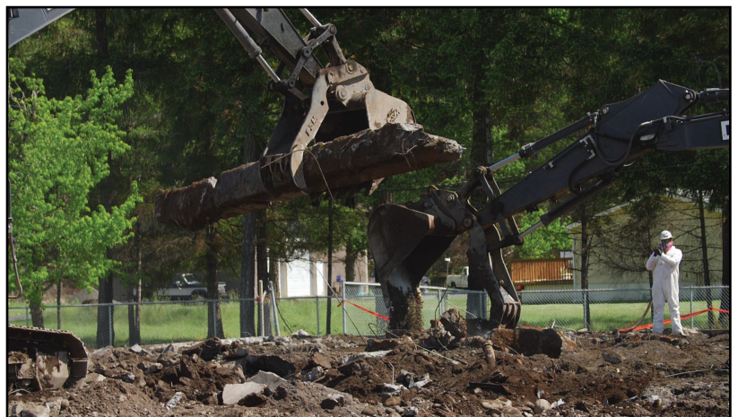
Ash and debris removal at Upward Bound Camp in Gates, OR
