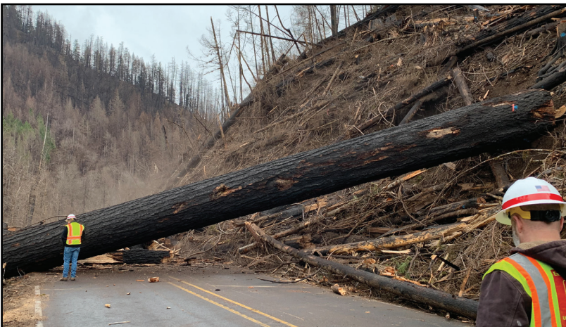
Crews assess fallen hazard tree on OR 224
